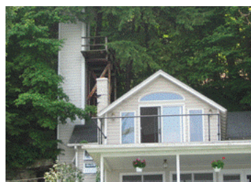
Lake house, Ithaca New York. The elevator shaft on the left created access from top parking to the entire house.
