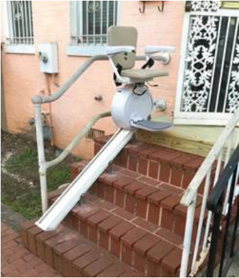
A wood platform at the top creates a zero-step entry at the doorway
